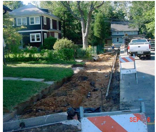
Project under construction
