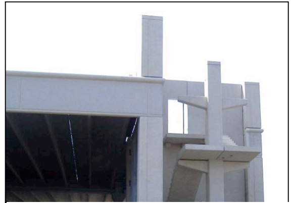
New parking deck under construction
