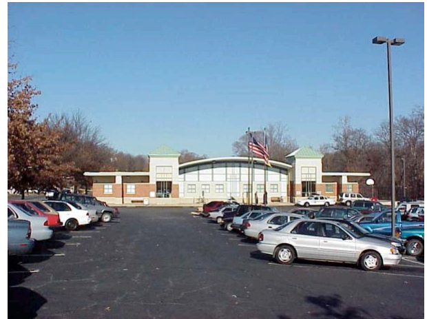
Existing Arlington Mill Community Center
