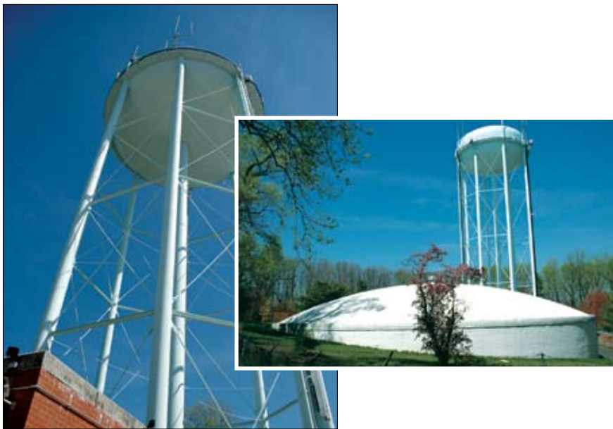
This water tower off Lee Highway holds a 30-foot deep elevated reservoir serving the higher elevations in north Arlington. When the water level drops below 25 feet, water from ground storage tanks (see inset photo) is pumped into the reservoir.
